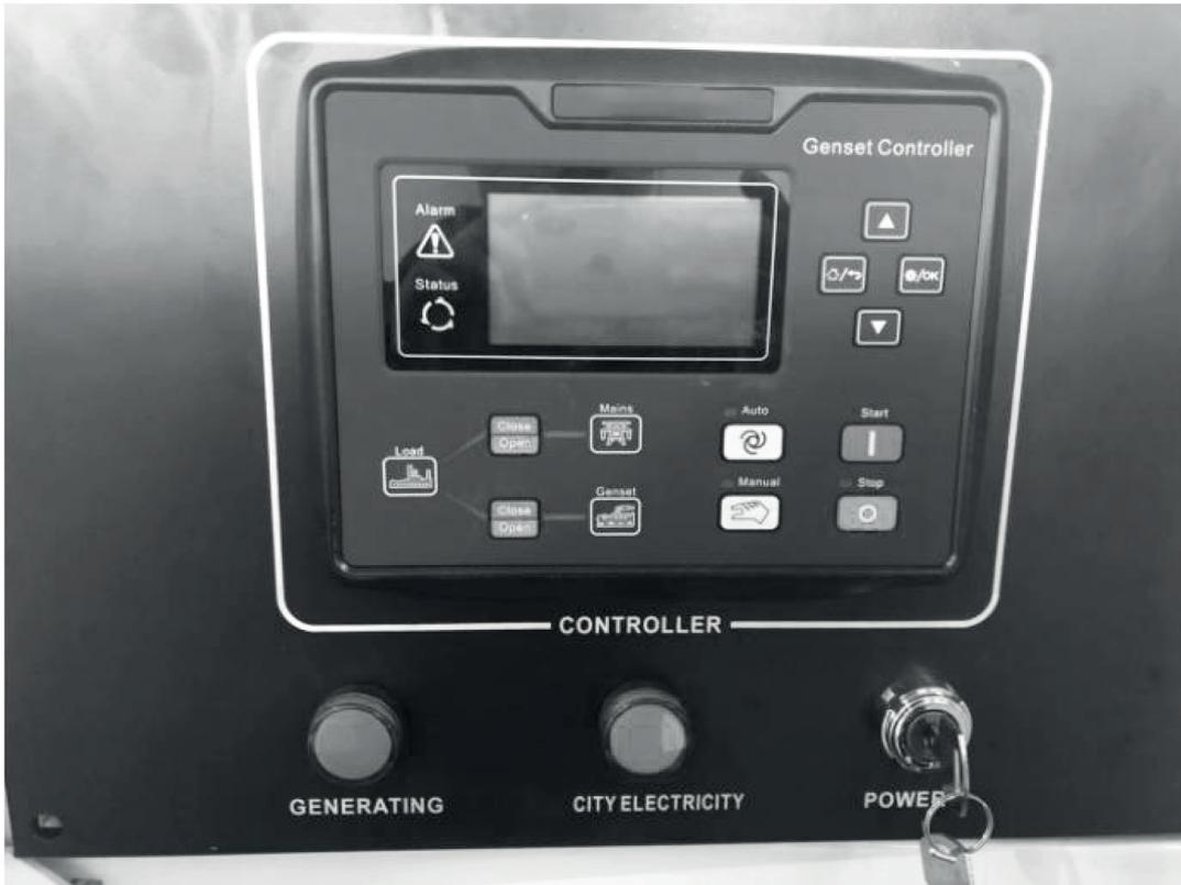
Final step: Finish set up the generator and then turn on breaker for auto protection
