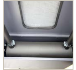
Residential muffler -35 dBA for enhance sound attenuation
